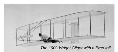
Will had added a fixed tail to the 1902 glider in hopes of avoiding this well-digging. There were two vertical panels of cotton muslin mounted on outriggers sticking out behind the wings. The panels did not move; they were not part of
